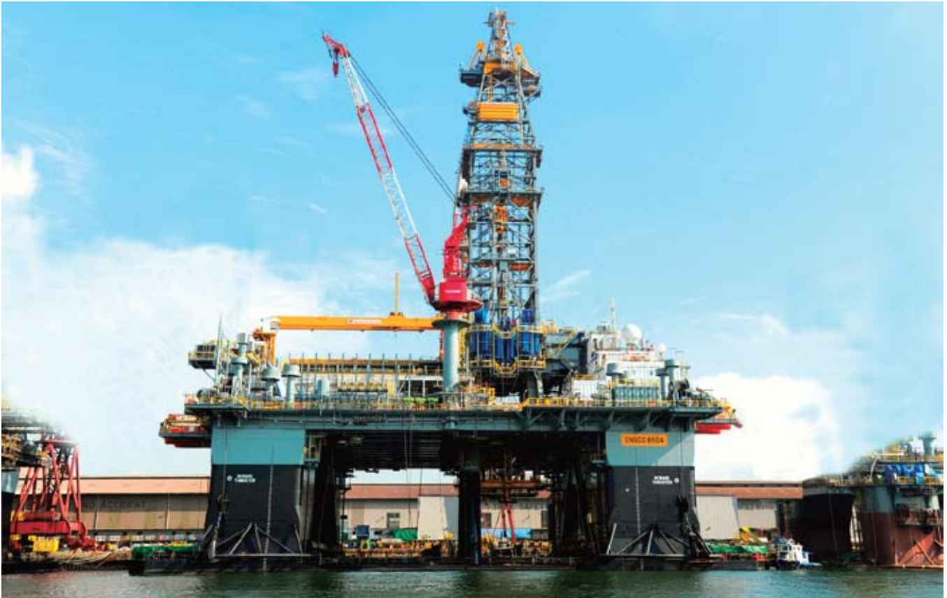
Delivered on time and on budget, ENSCO 8504 is the fifth of seven ENSCO 8500 Series® ultra-deepwater semisubmersible drilling rigs Keppel is building exclusively for Ensco
